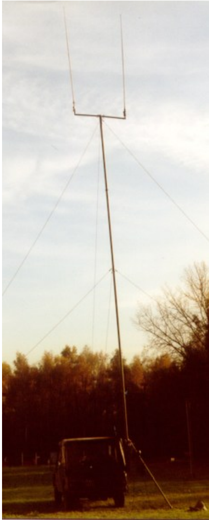
2 antennas on ULM-11/QESH mast
