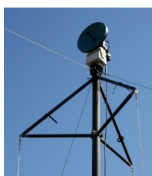
Anti-twist systems Star-Bar and T-Bar
